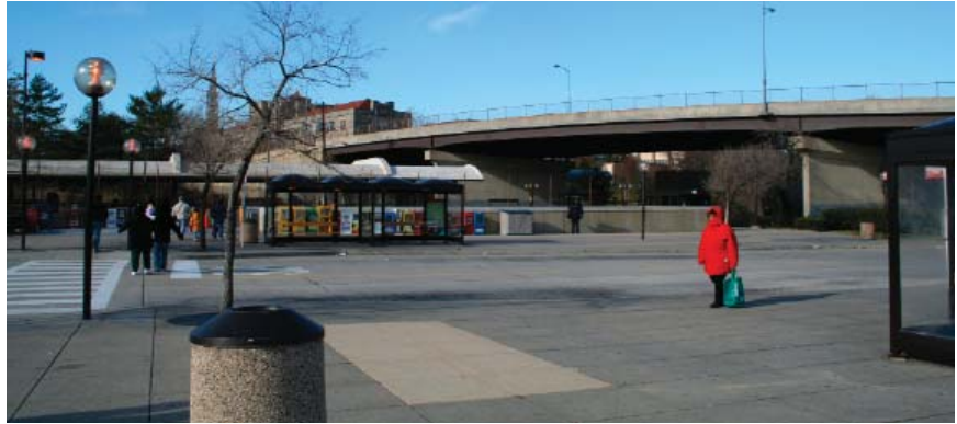
Brookland/CUA Metro Station entrance from the east
