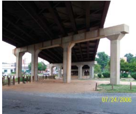
Area under Michigan Avenue bridge
