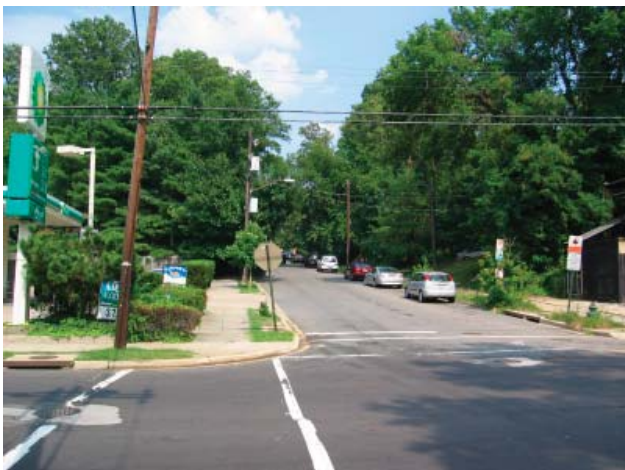
Poorly marked crosswalks – Otis at 12 th Street
