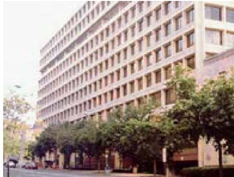
Connecting Downtown with Downtown East will expand the commercial core eastward to Union Station, rather than to Shaw.
