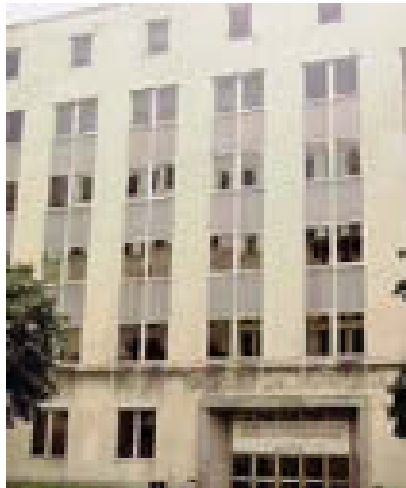
With proper funding initiatives, publicly owned sites (like the DOES building above) can be maximized.
